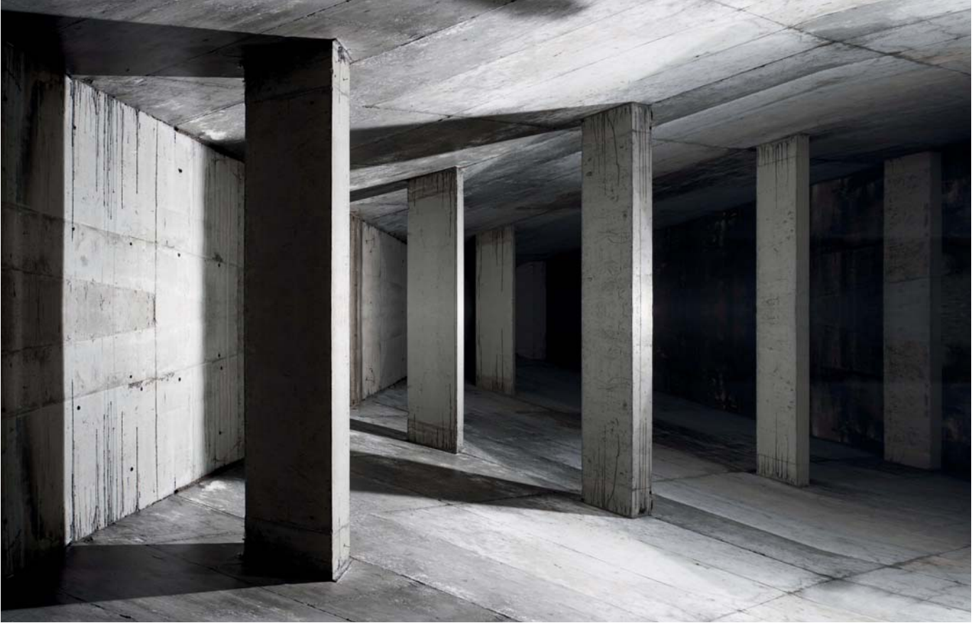
Landscape Under Construction Alfonso Batalla
